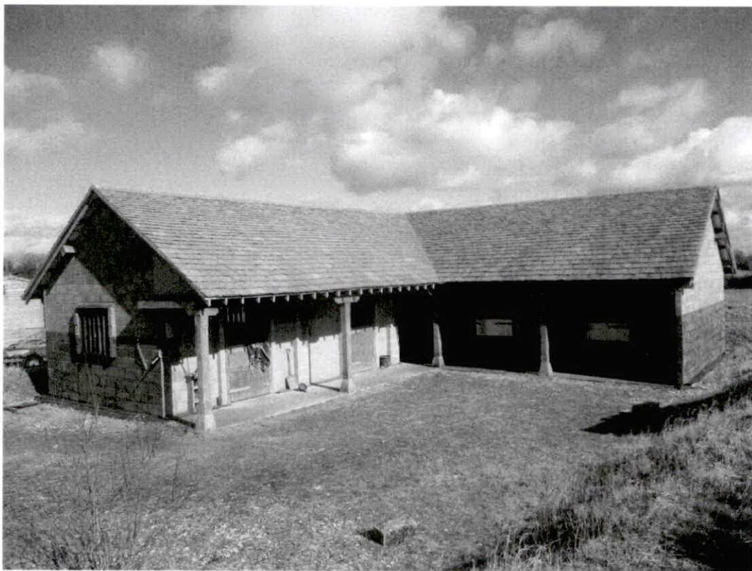
Below: Existing building
